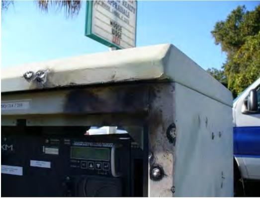
*Thankfully, I was wrong. Throughout the entire ordeal our power supply equipment continued to operate keeping the cable system online. Our power supplies did switch over to standby mode once the power company's fuse finally opened and commercial power was lost to our equipment. During this event the cable system never failed to keep operating.*
